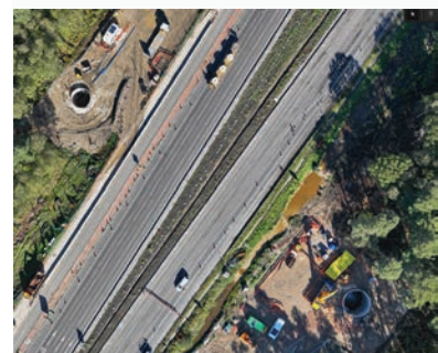
Aerial view of drill sites either side of the carriageway
