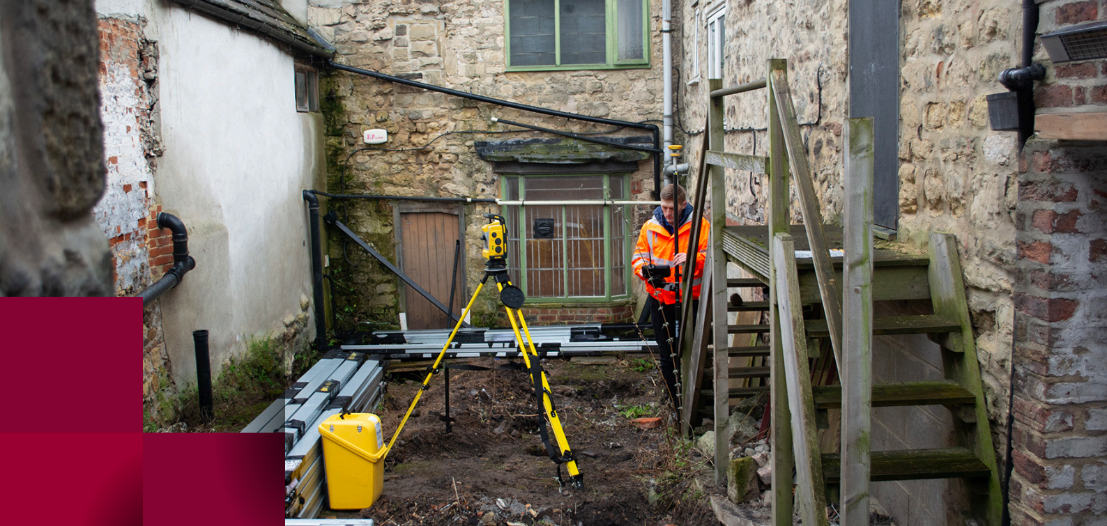
Just 20 minutes to set out the screw pin foundations using a Trimble Total Station
