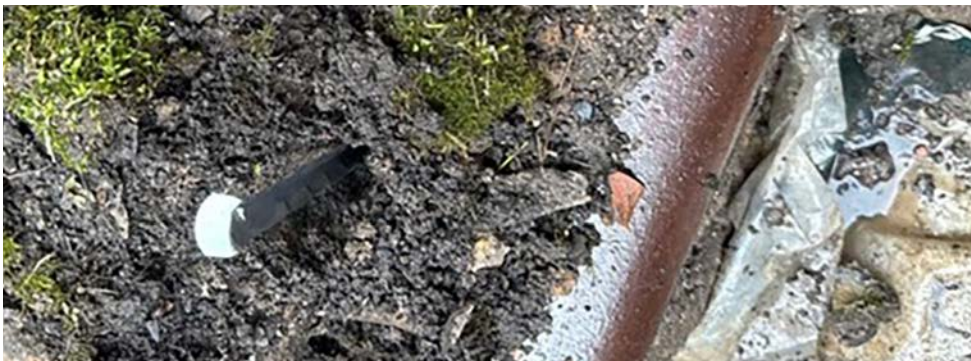
Showing how one of the screw pins would strike a service. The setting out allowed Stephen to conduct calculations and assess that this service needed to be relocated away from the pin location
