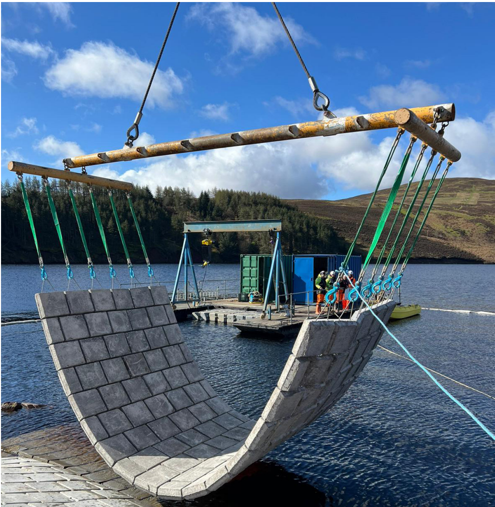
Positioning of flexible concrete mat prior to pipe installation
