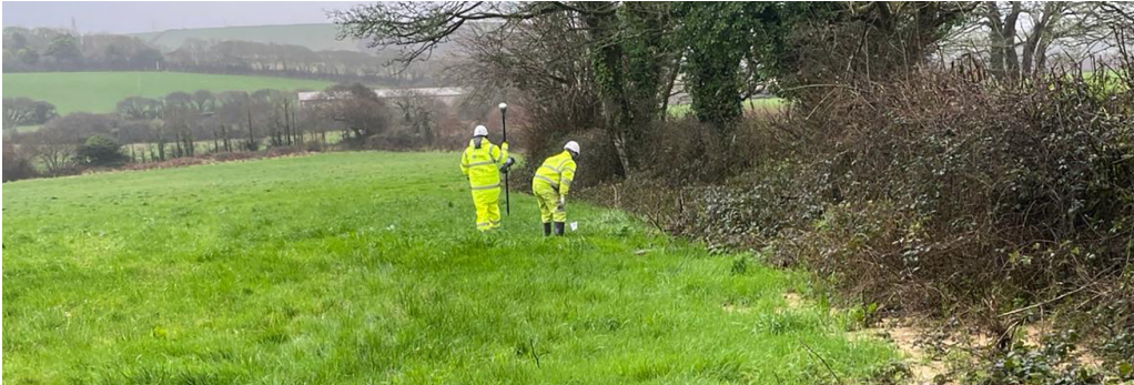
The R12i was used extensively across the project for topo, control and setting out the Cornish hedges
