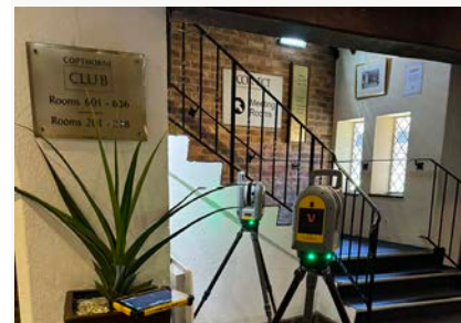
The stair core was scanned to see how the floors align in a hotel
