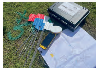
Ready for site set out
