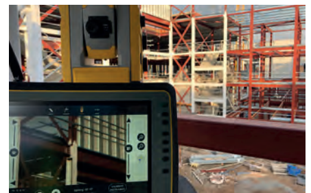
▲ Trimble FieldLink running on the Kenai tablet
