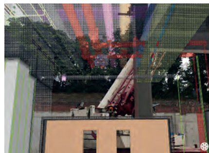
▲ Image taken from Dalux showing the services set out in augmented reality
