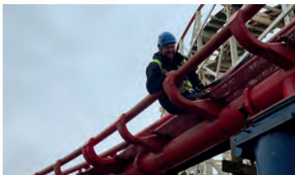
▲ Jake Roper-Fairhurst placing retro targets
