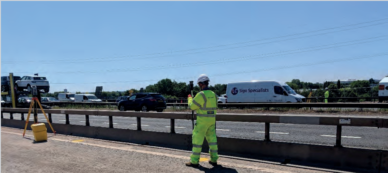
▲ Setting out superspan gantries from both northbound and southbound
