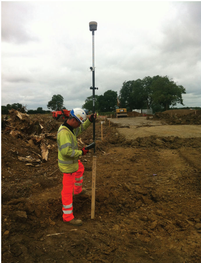
▲ Skanska on the M1 site with the R10 – no need to look at the pole to check its level thanks to the eBubble facility on the TSC3 logger
