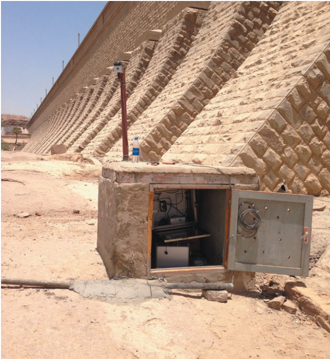
Old Dam Free Field Station
