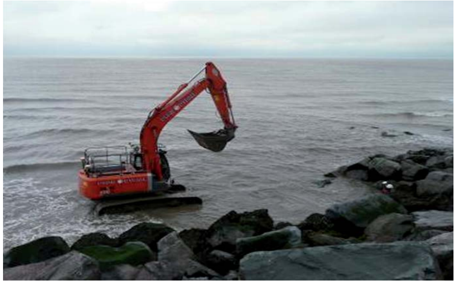
▲ Trimble GCS900 system mounted on Dean & Dyball’s Hitachi ZX250 excavator
