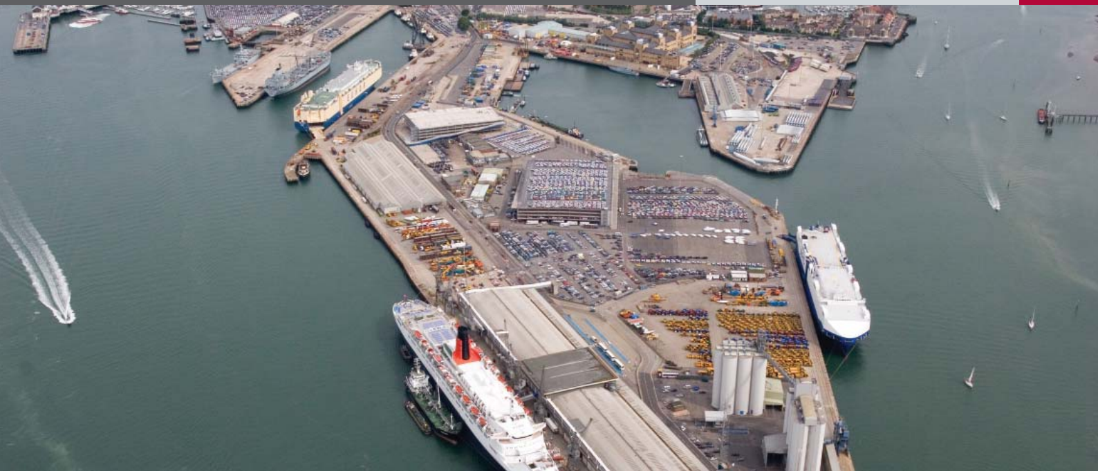
▲ Southampton Port Aerial View
