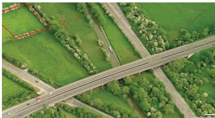
▲ An aerial view of the old viaduct built in 1961
