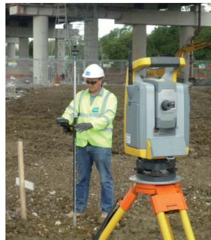
▲ S6 being used to reset the earthworks profile
