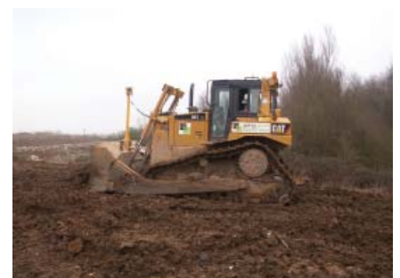
▲ Trimble GCS900 system on Going Green Restoration’s CAT D6T dozer
