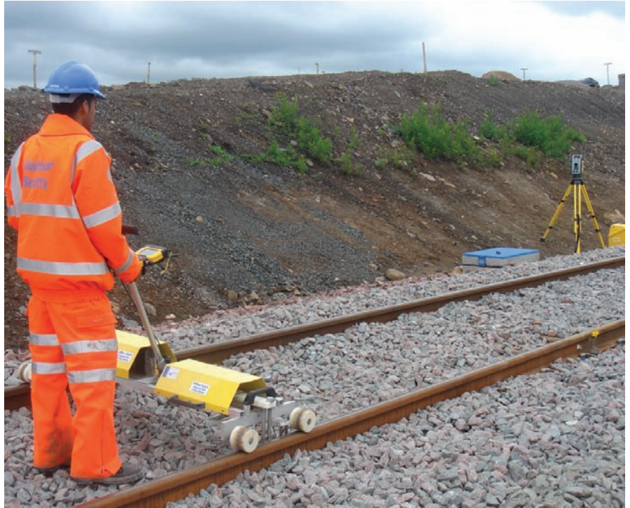
▲ The TMD on site between Bathgate and Airdrie
