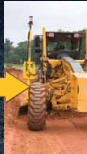
Bulk Earthworks to Fine Trimble GCS900 Grade Control
