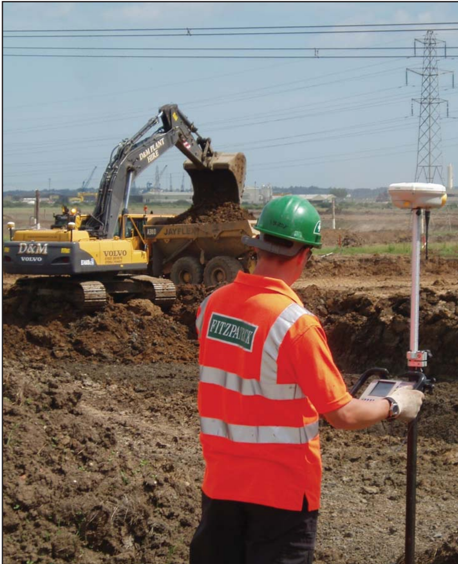
Mark Humphrey checks work done with a Trimble Rover and ACU logger
