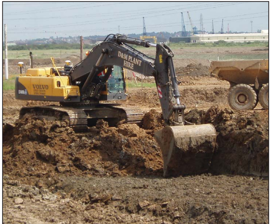
The Trimble GCS900 mounted on a D&M Plant Volvo EC460-GC
