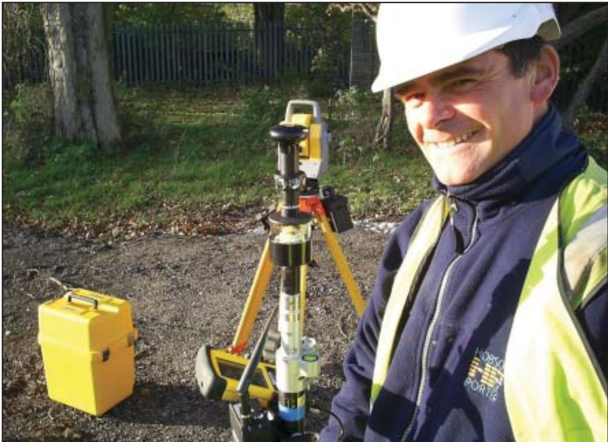
Spot on! Paul Hostick out on site with Trimble's LM80 Layout Manager and 5600 Robotic Total Station
